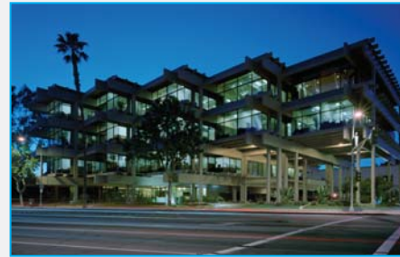
Warner Bros.' LEED™ Silver certified green building is the first in the industry.
